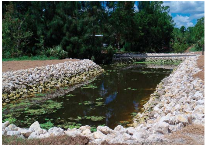
Canal 3 extension to Riverbend Park
