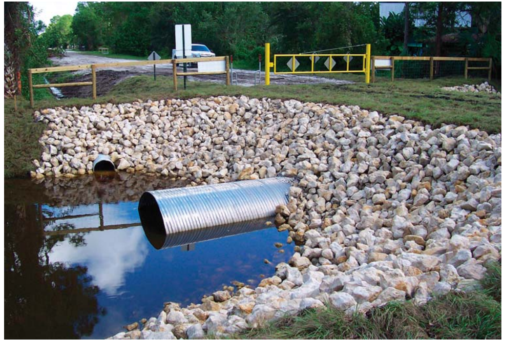
Culvert and embankment improvements at Canal 7 and Alexander Run
