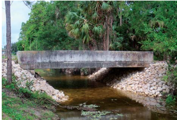
Canal 2/Hatcher Bridge embankment restorations
